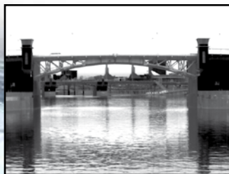
Burnside Bridge, Thermal image
